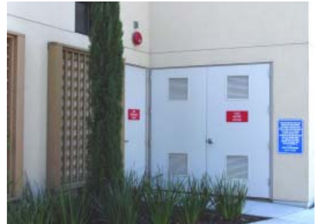
Utilities enclosed in building.
