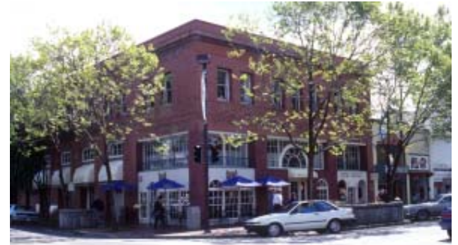
Windows and awnings delineate ground floor storefront.
