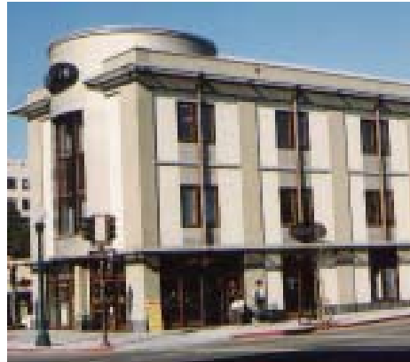
Building with multiple ground floor entries.
